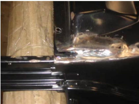
Figure 4. Steel overlap welded on the window frame.
